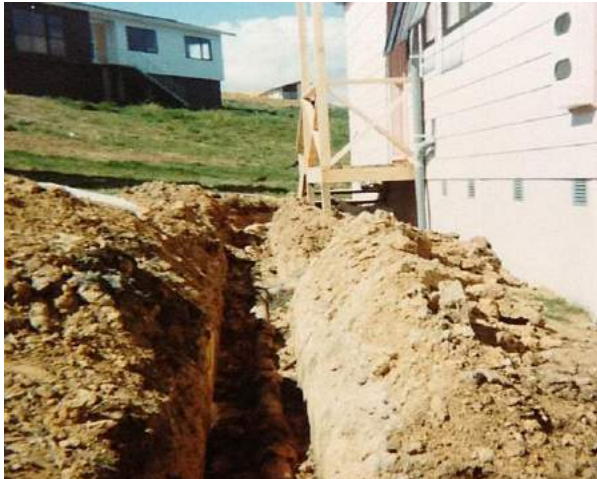
To save money I dug the drains (by hand!)
