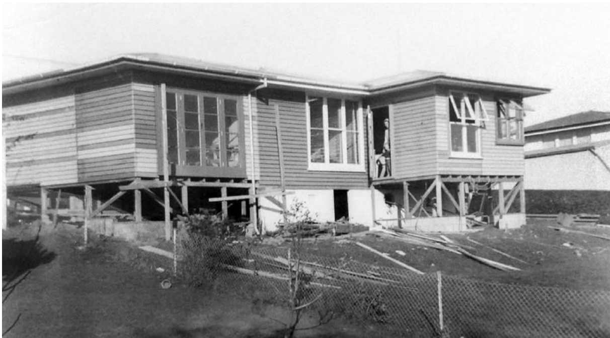
The renovations at No. 9 Farrington St
