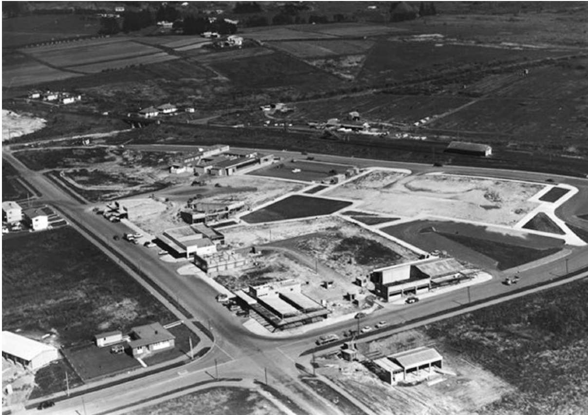
the Glen Innes shopping centre being built 1960
