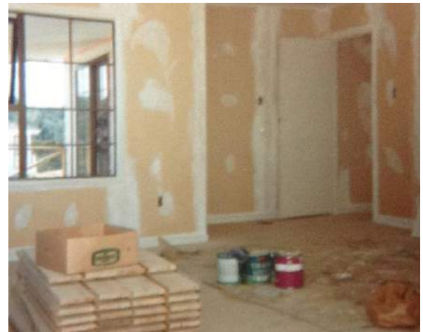
The plastering complete!
