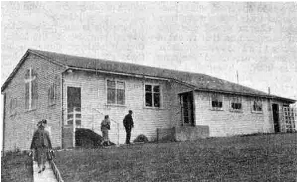
St Timothy's Church in 1956 before the addition of the Langley Block
